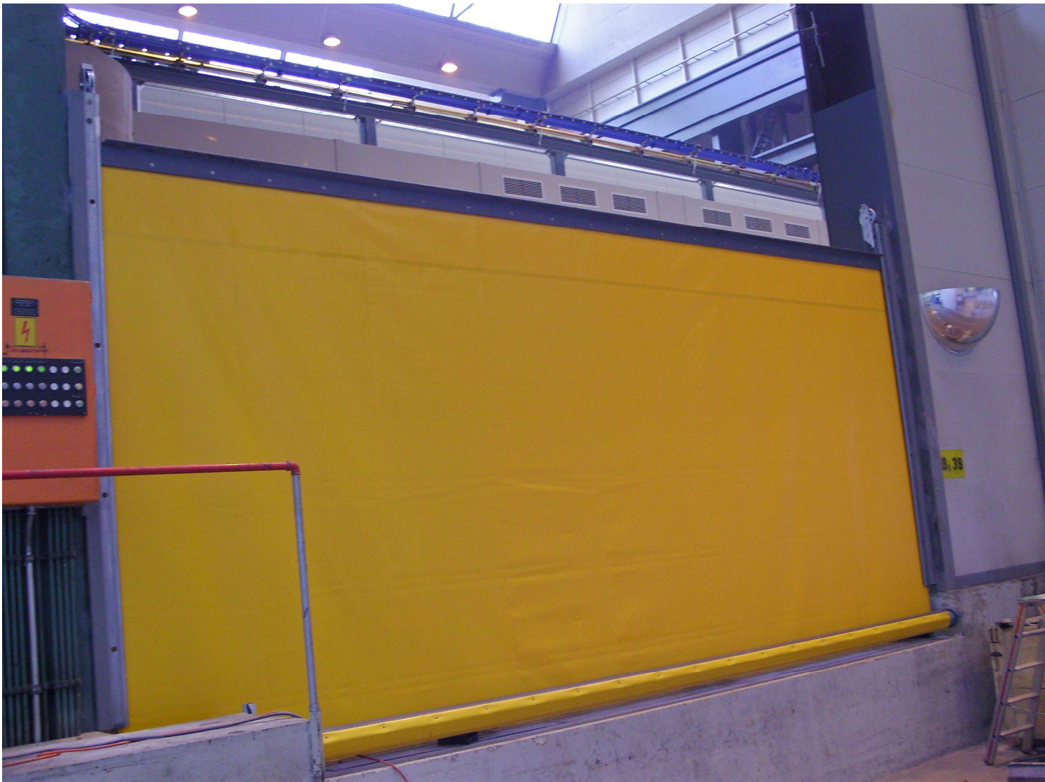
Roller Door with turning tube and drive unit down below floor level
